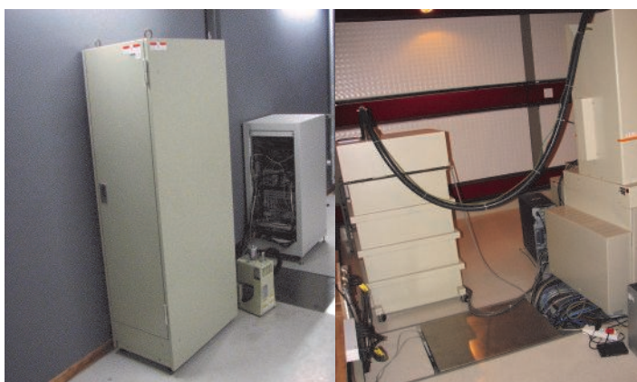
All vacuum pumps, water chillers and compressors are housed in the buffer rooms. To minimize electrical and noise disturbances, all electrical wires are neatly tucked beneath the floor panels and acoustic tiles have been fitted against the walls.
