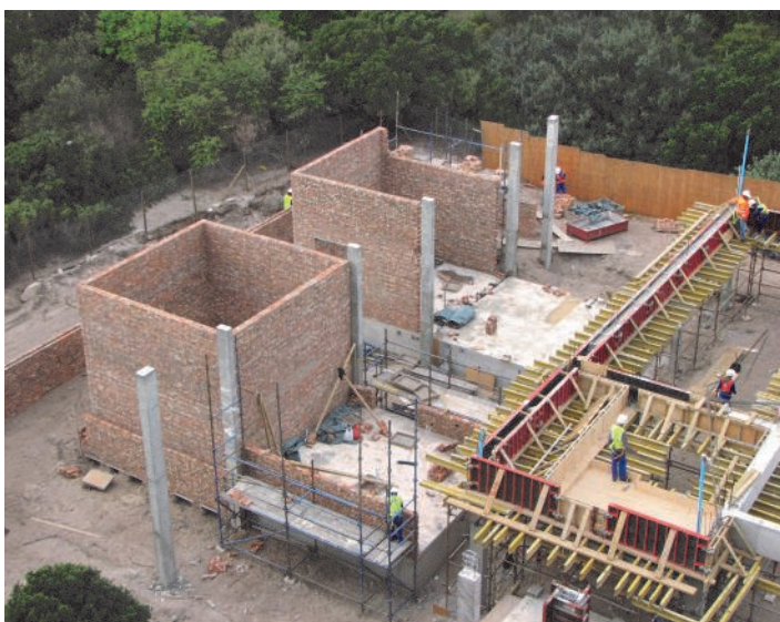
Construction of the four microscope rooms that are isolated from the main building.
